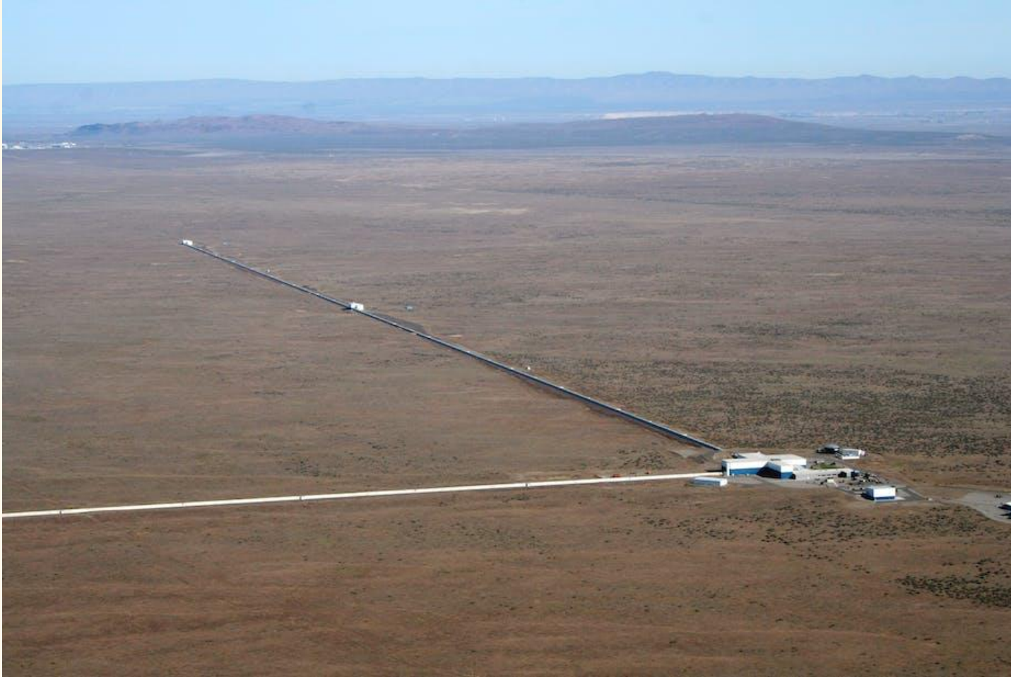
The 4km long arms of the LIGO experiment at Hanford. LIGO lab: www.ligo.caltech.edu
